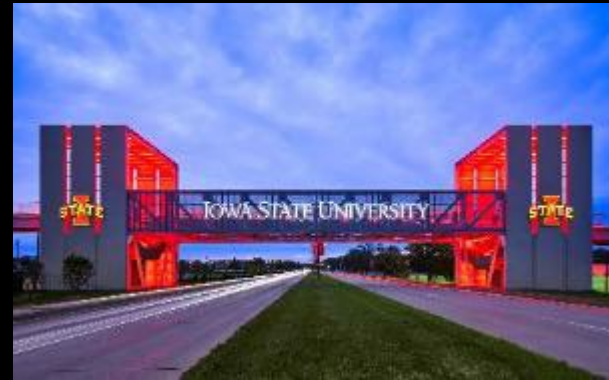
Iowa State University East Gateway Pedestrian Bridge / Ames, IA
