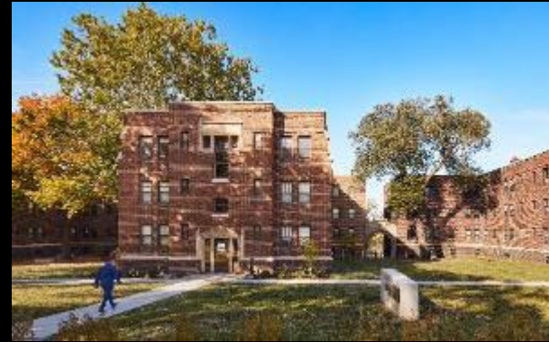
The Tree House Apartments Renovation / Des Moines, IA
