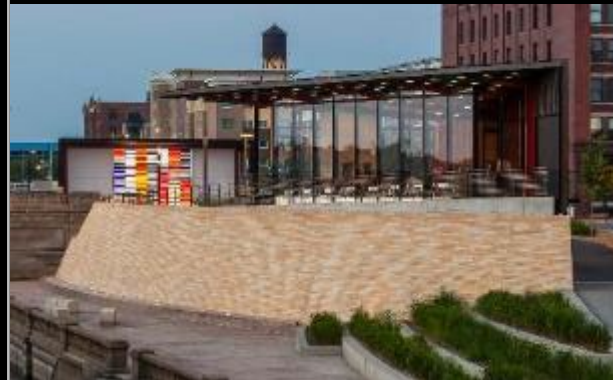
Principal Riverwalk Pavilion and Pump Station / Des Moines, IA
